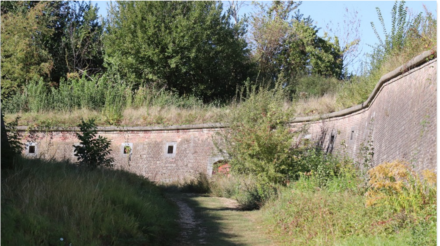
Fig 9. View on the northern- and western wall during the morning.
