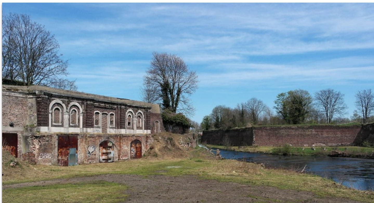
Fig 20. View of the wet moat (and former harbor) Havenkom with remnants of the Lage Fronten fortifications (11-04-2016). To the left Casemate Ravelijn A, and to the right Bastion B. (Source: KLEON3 at Wikimedia Commons).
