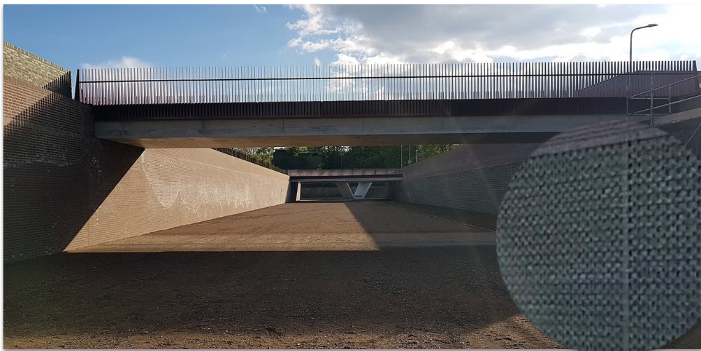
Fig 14. Cabergerweg underpass, with detail of the lizard-friendly wall (28-04-2019). (Source: KLEON3 at Wikimedia Commons).
