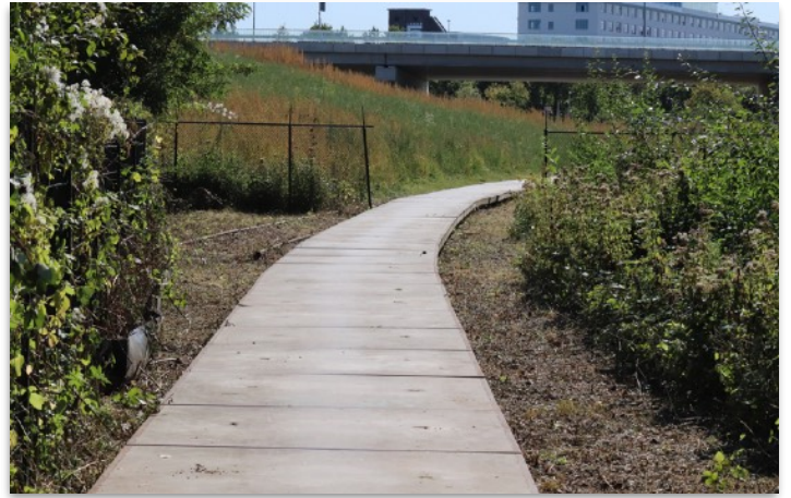
Fig 28. Concrete footpath with two lizards “visible”.
