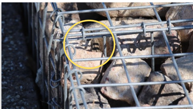
Fig 23. The stone baskets are being used (Lage Fronten).
